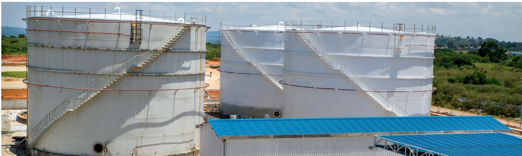
Grain storage silos © OPM
